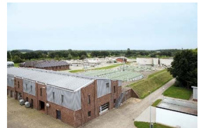
Edeweicht wastewater treatment plant
